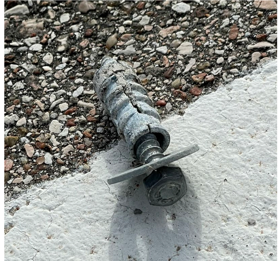
Photo of Concrete Anchors Laying in Parking Lot
