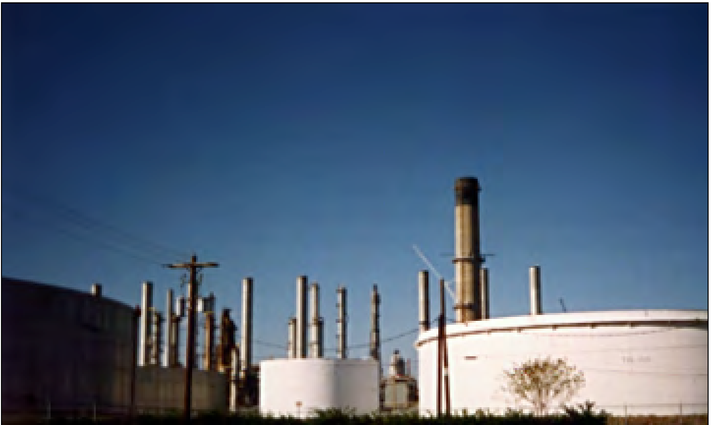
Petrochemical plants are part of the Harris County environment.
