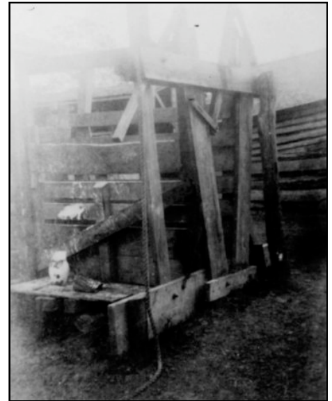
Butler constructed a series of loading chutes that permitted the simultaneous loading, or unloading, of four cattle cars on the adjacent railroad siding.
