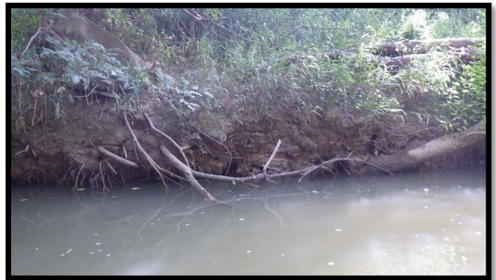
Figure 32 View of left bank taken from transect 3 during critical period.
