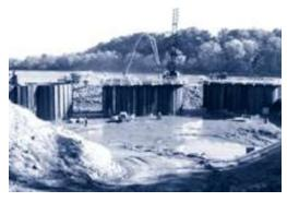
Crews erect coffer dam cells as part of the fish passage facility at York Haven, Fall 1998. The construction will be complete in time for the spring shod run in 2000.
